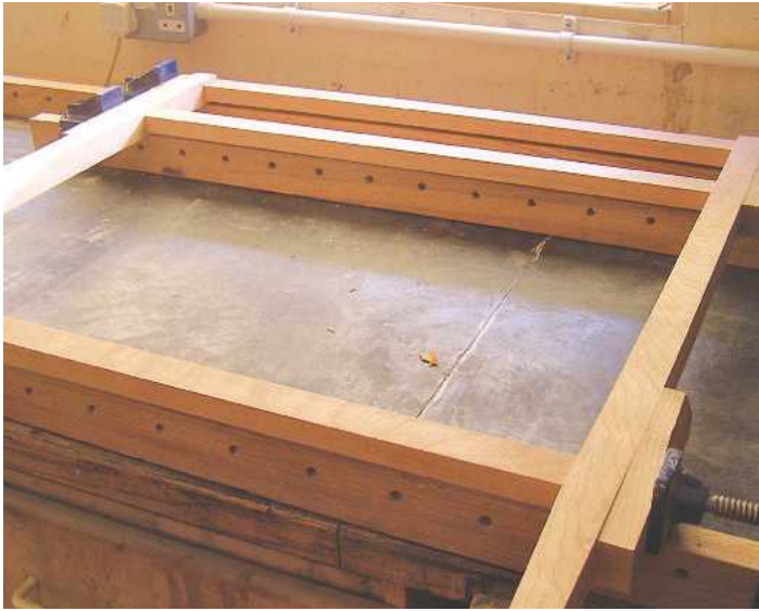
▲ Pic.8 Having cut the joints, glue the front and rear frames together, being careful to ensure squareness
